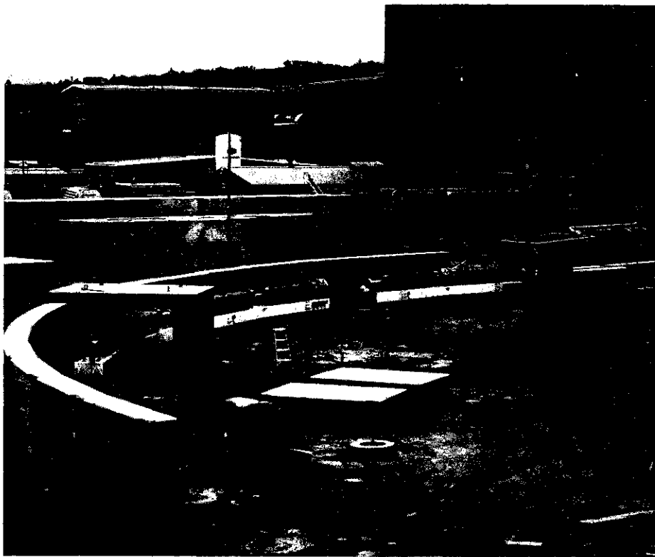
Benefiting from the splendid Californian climate the electron-positron storage ring SPEAR takes shape in the open air near the output end of the 20 GeV electron linear accelerator at Stanford. First tests with the completed ring are scheduled to take place early summer next year.
